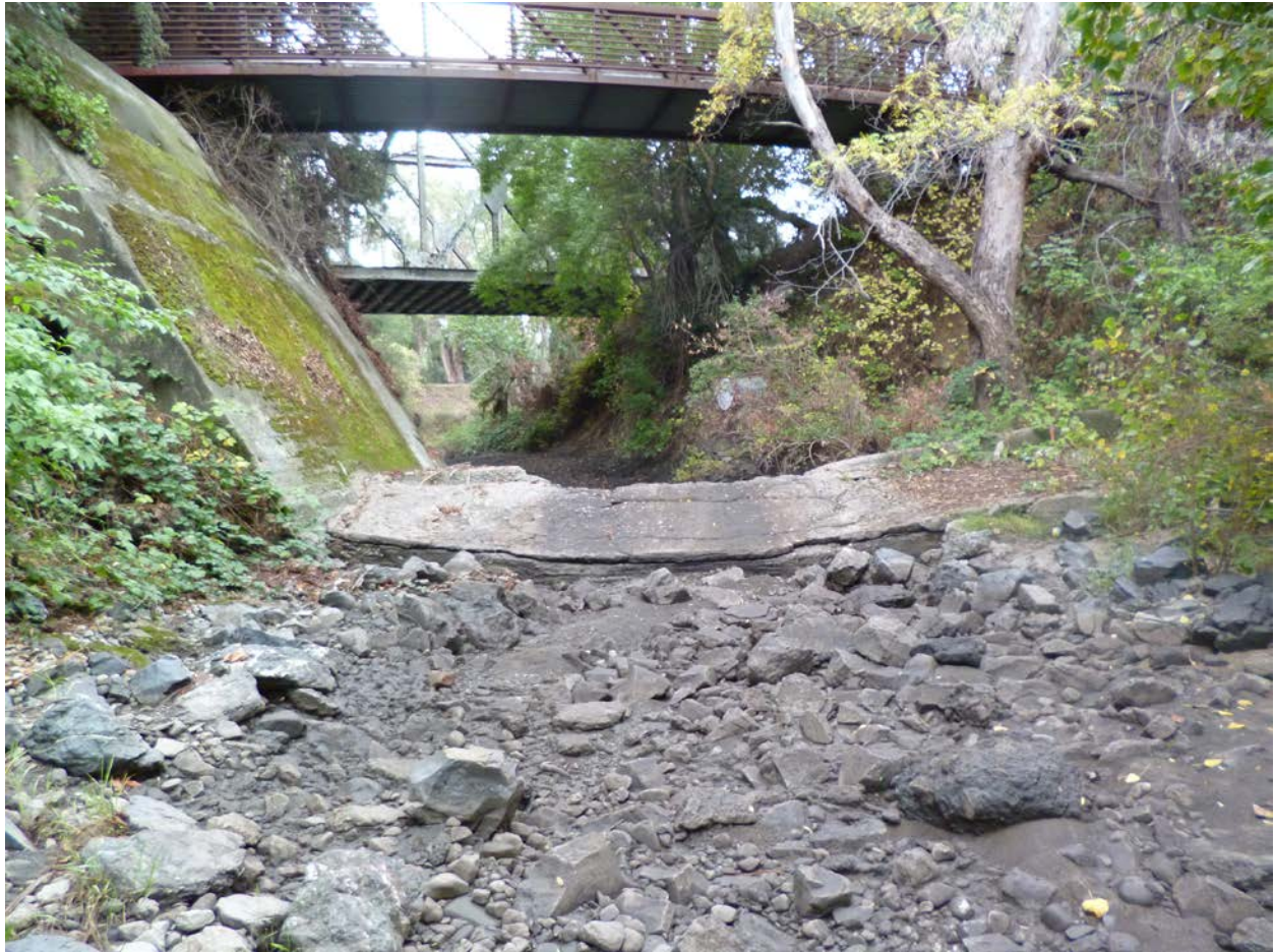
Figure 2: Bonde Weir looking from downstream to upstream.
