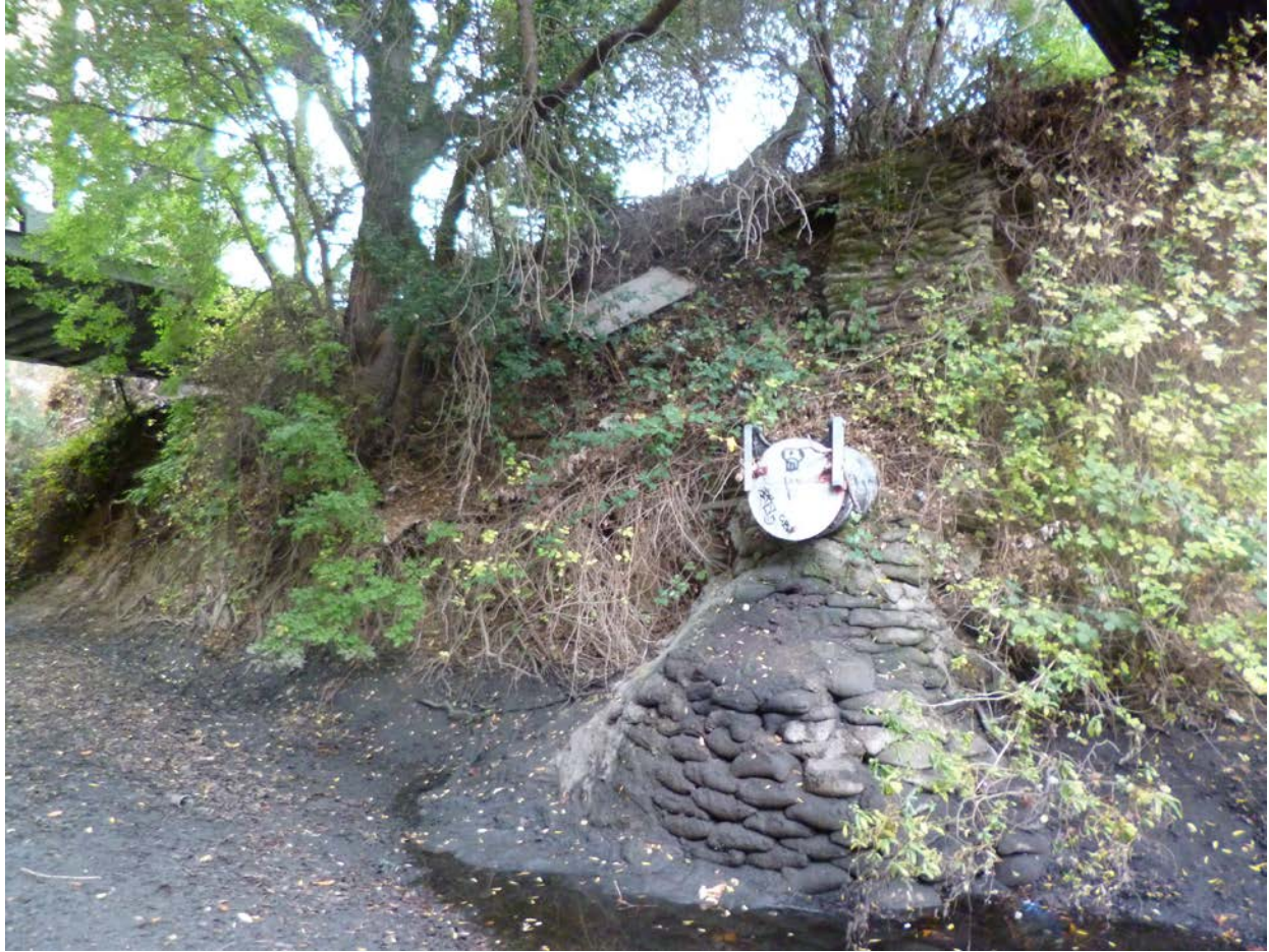
Figure 5: Storm drain outfall on the left bank just upstream from Bonde Weir.
