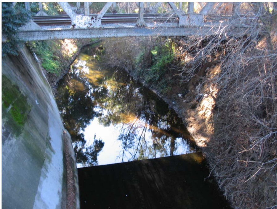
Figure 2-2: San Francisquito Creek Upstream of the Alma St Pedestrian Bridge
