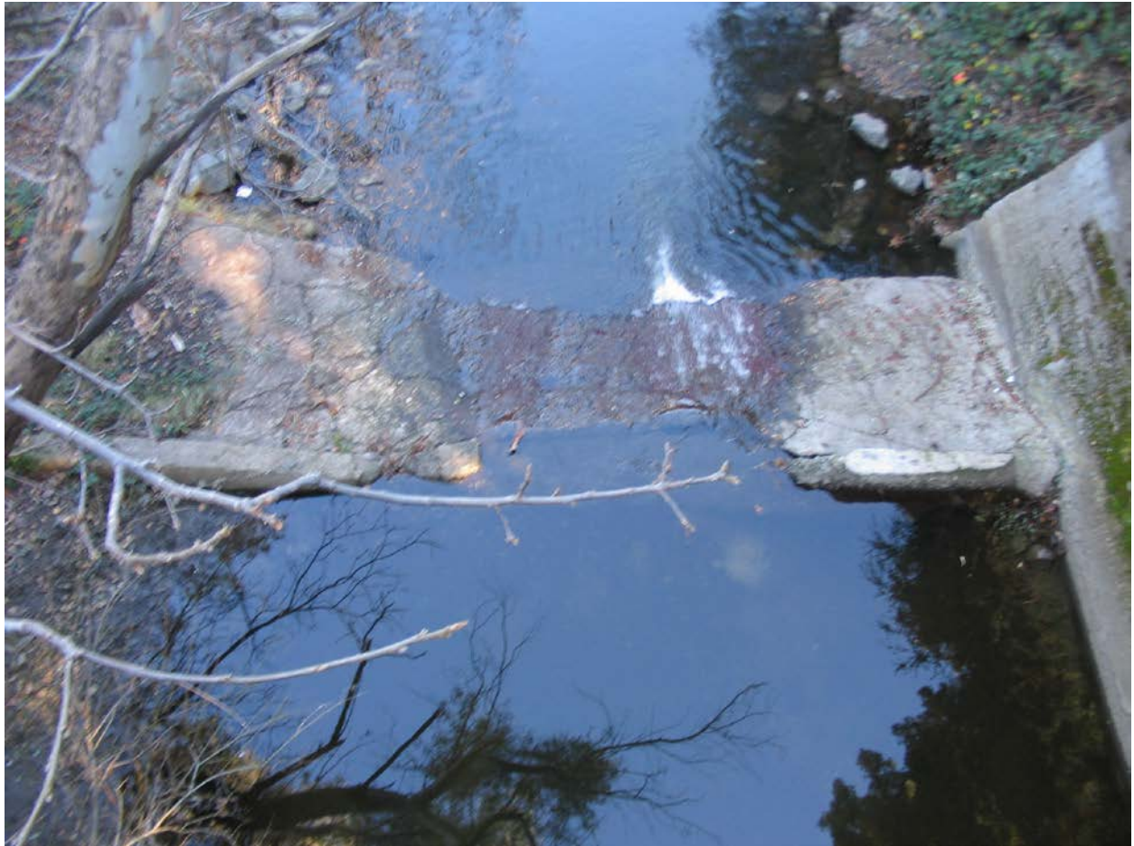
Figure 4: Bonde Weir looking from upstream to downstream from the pedestrian bridge above.
