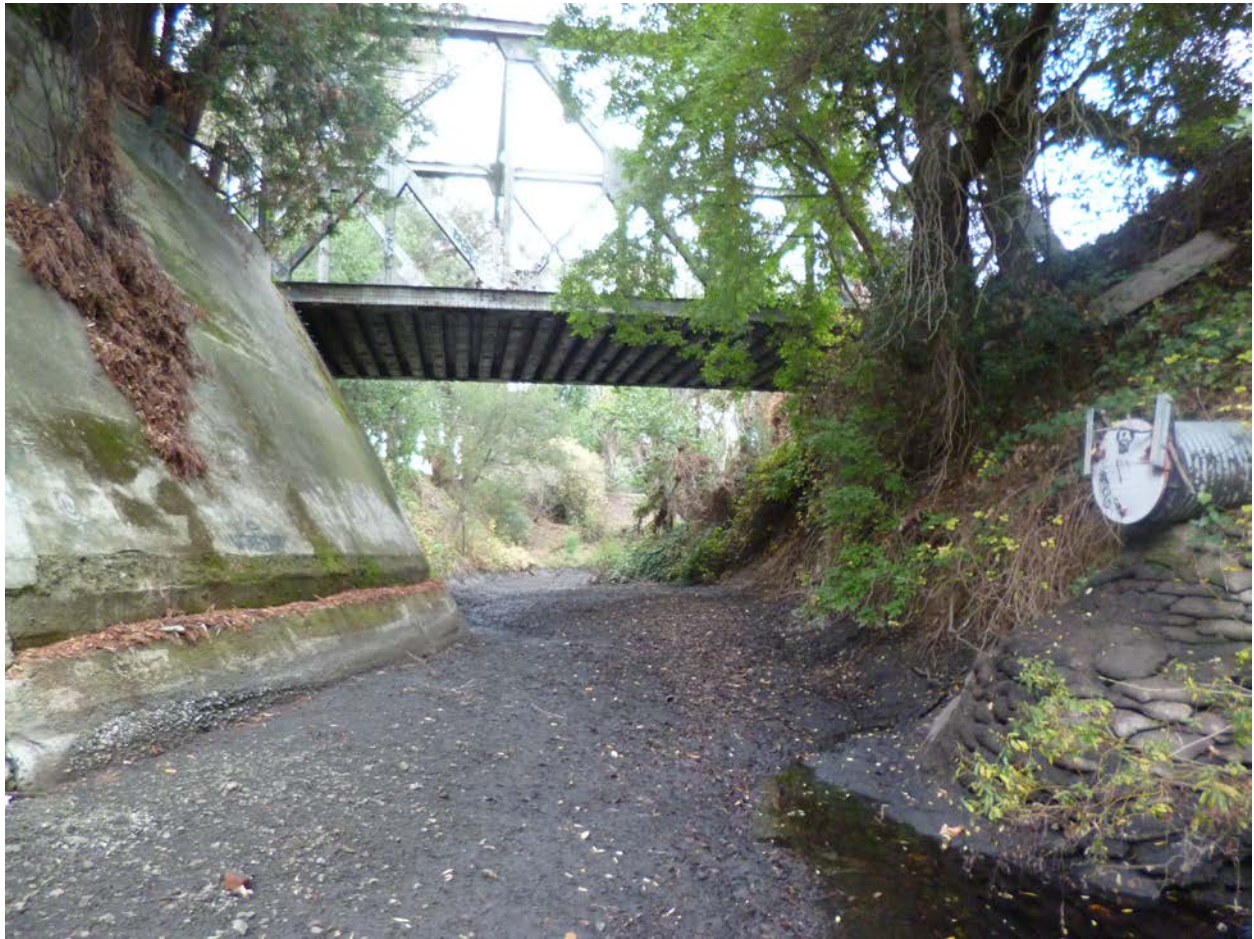
Figure 1: Looking Upstream from Bonde Weir.
