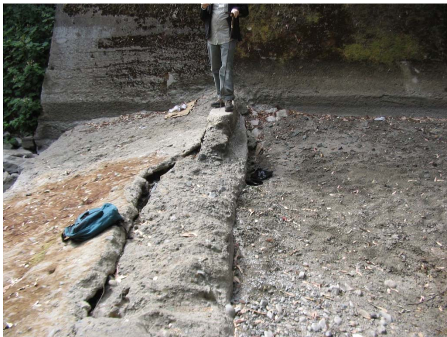
Figure 2-4: Bonde Weir Crest
