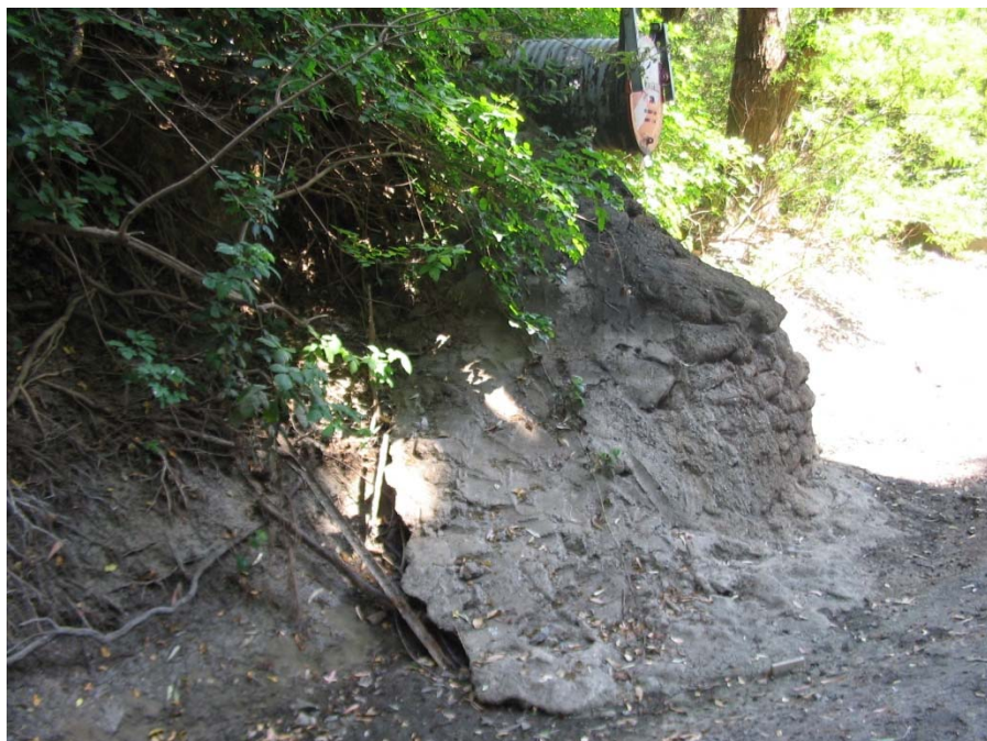
Figure 2-6: Bonde Weir and Storm Drain Outlet
