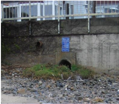
Capistrano Outfall Pipe
