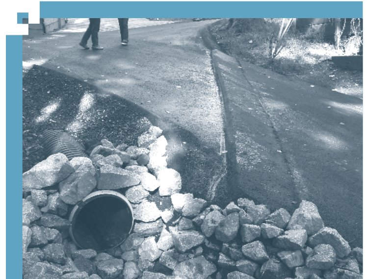
Figure 10. Asphalt waterbar and culvert outlet, both with rock dissipater to reduce erosion.
