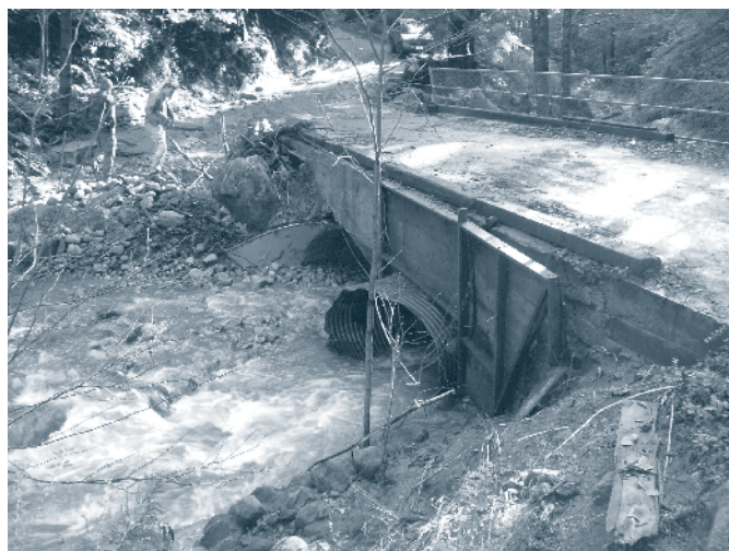
Figure 26. Failing culverts were a safety hazard and the crossing flooded during large storm events. The rusted culverts were impeding fish passage.
