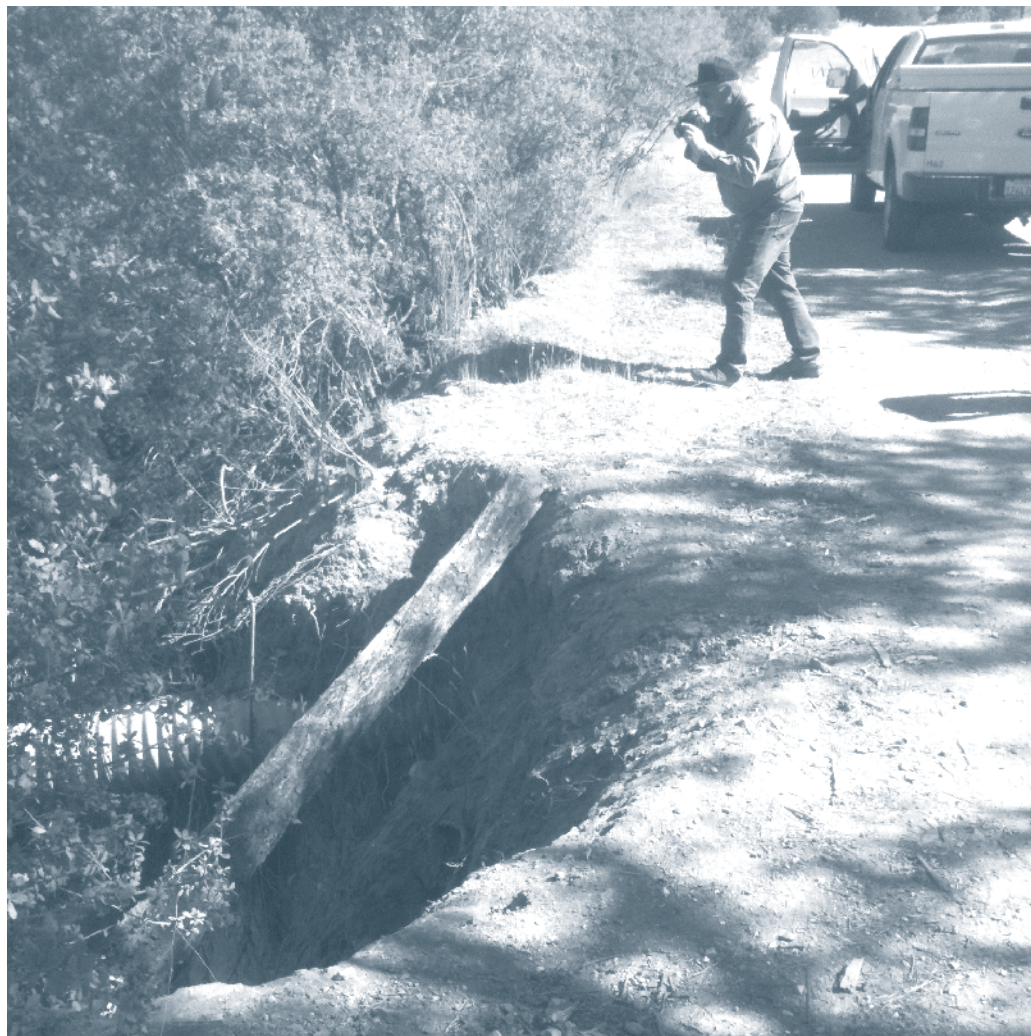
Figure 5. This road washout is the result of an undersized and improperly placed culvert.
