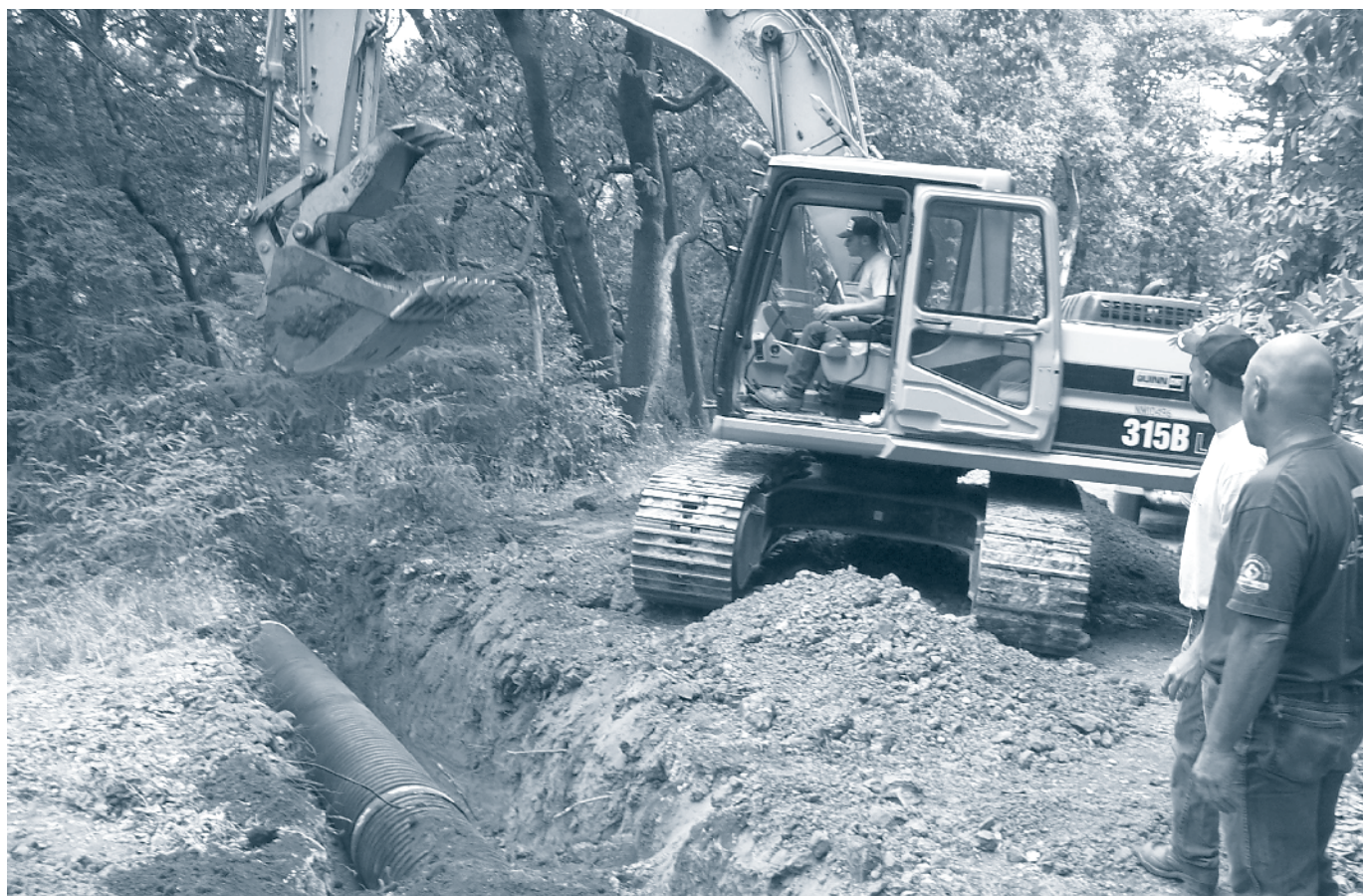
Figure 28. The culvert installation included proper angle placement and was back filled and compacted to design specifications.
