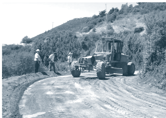
Figure 22. Road grading.
